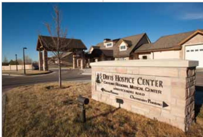
Davis Hospice Center, Cheyenne Regional Medical Center
