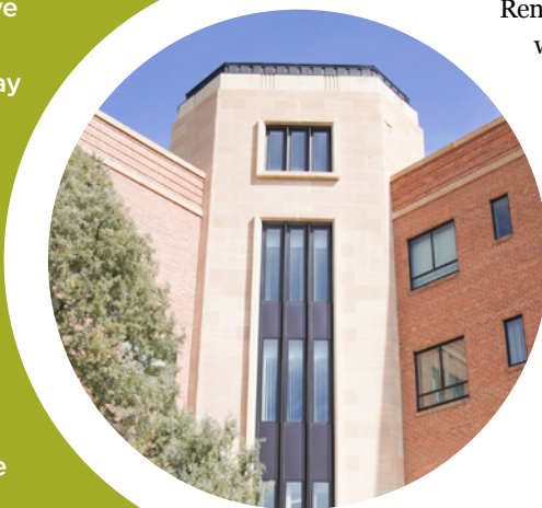
A detail of the exterior of CRMC East building, or formerly DePaul Hospital.
